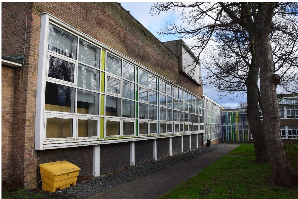
Photograph 5: Workshops (north end of Block E), looking south-east
