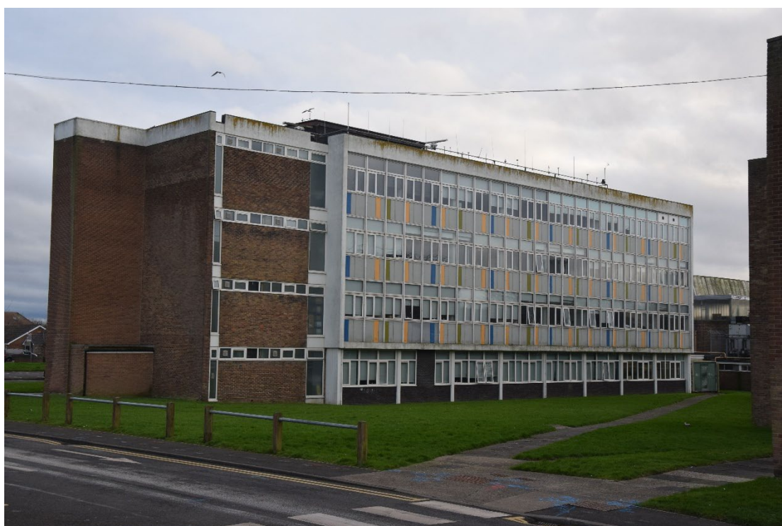
Photograph 24: Engineering and Navigation Department (Block G), looking south-west
