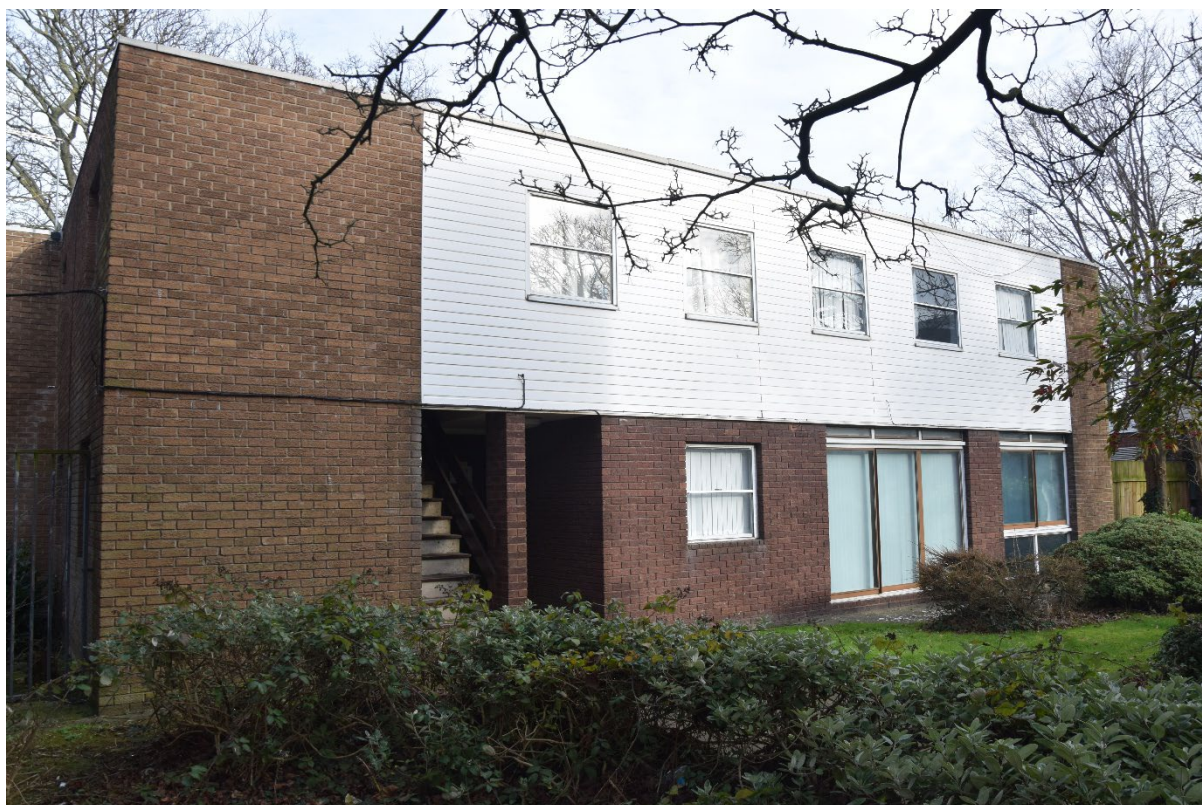
Photograph 37: Accommodation block, looking north
