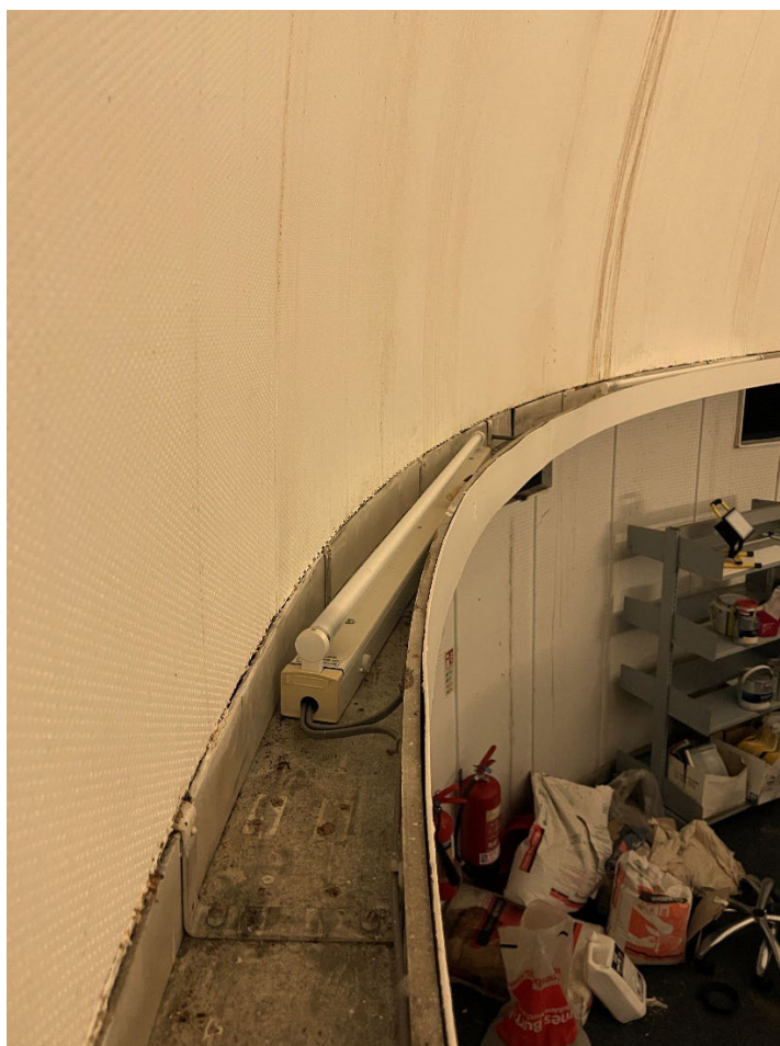
Photograph 53 (left): Gutter around the internal edge of the planetarium dome for fluorescent tube lighting, looking east
