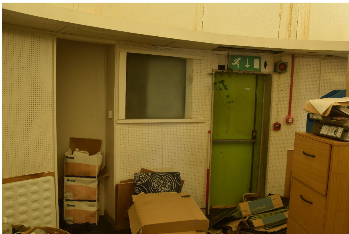
Photograph 59: Fire escape door on the south side of the planetarium, looking south
