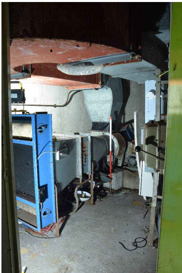
Photograph 47 (left): Plant room, looking east
