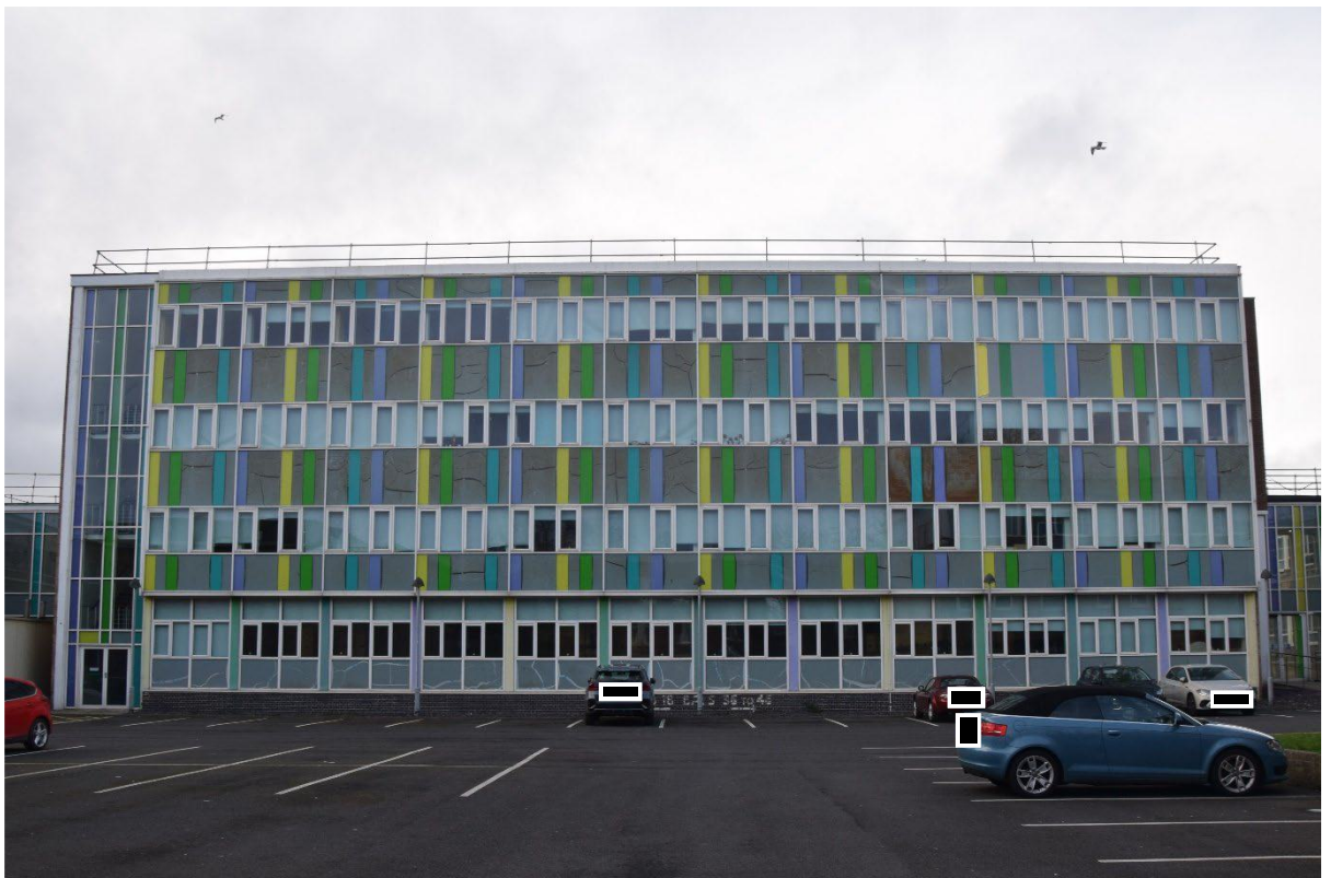
Photograph 18: The Commerce and Art Department (Block D), looking north-west
