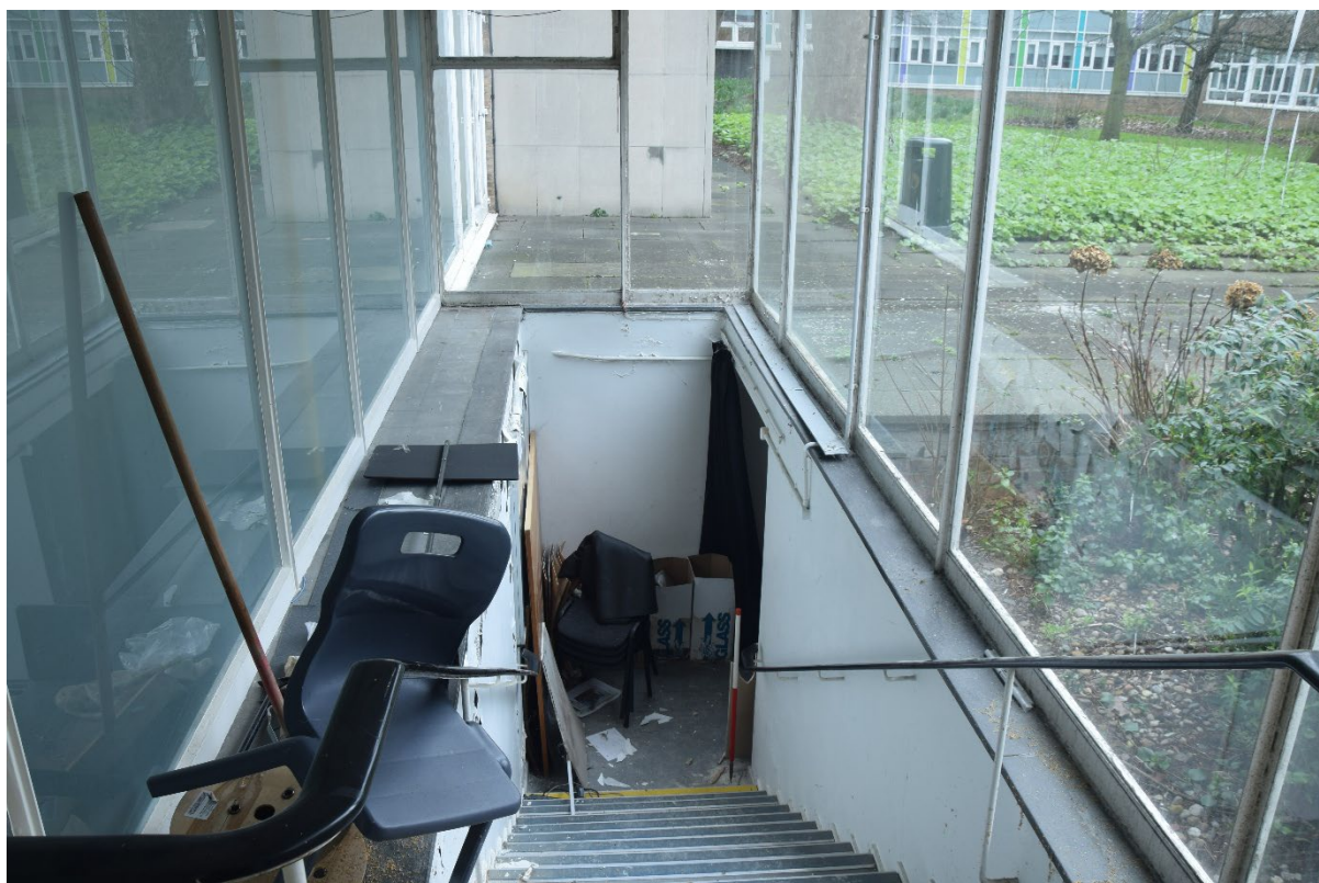
Photograph 45: Atrium staircase, looking east
