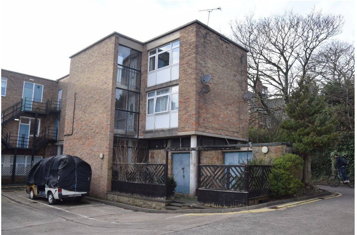
Photograph 17: Accommodation block attached to the Women's Work Department (north side of Block B), looking west
