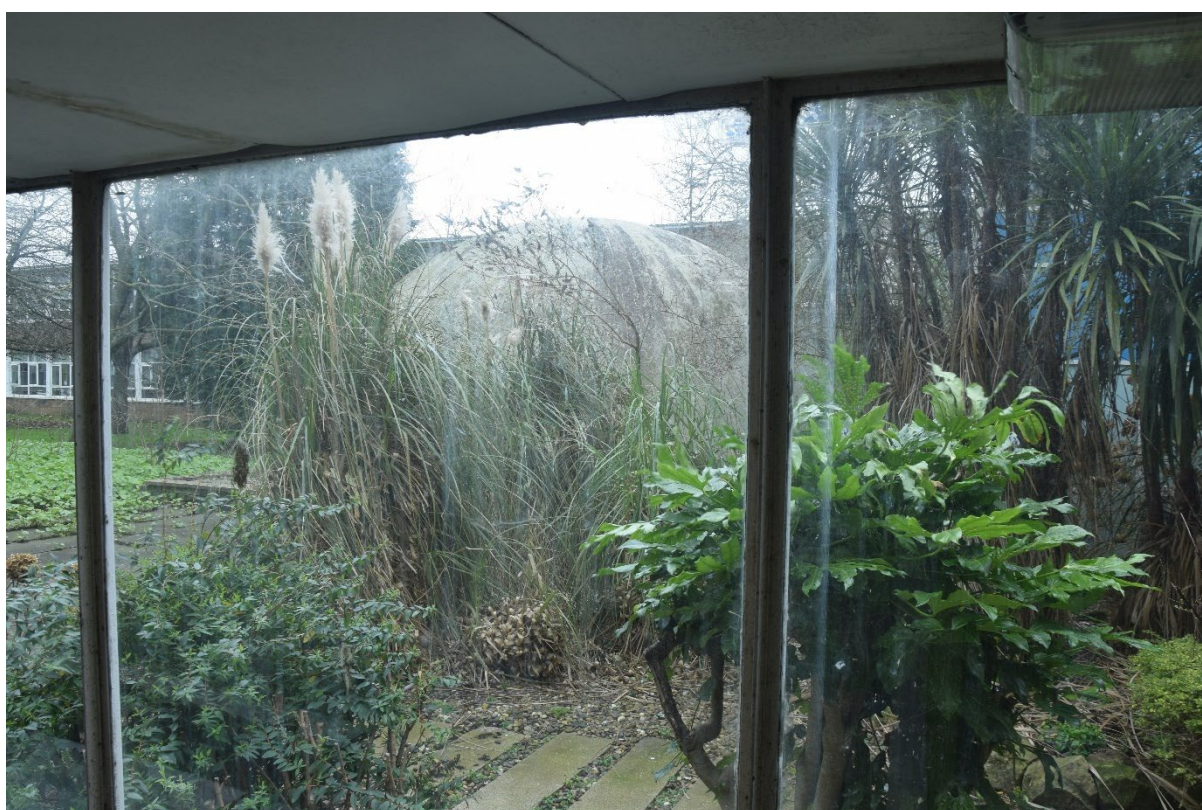
Photograph 44: View of the planetarium dome from the atrium, looking south-east
