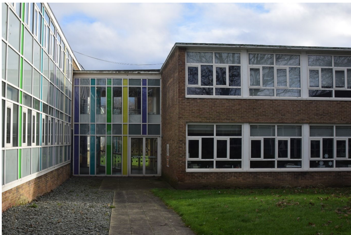
Photograph 11: East end of the Navigation Department (east end of Block C) with link to the building department and workshops, looking south-east
