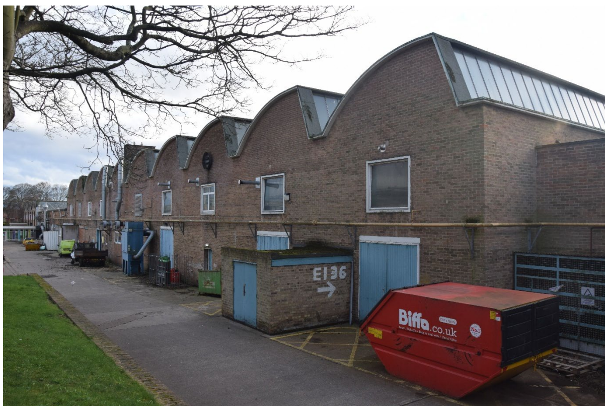
Photograph 6: Workshops (Block E), looking south. Note the sawtooth roofline.
