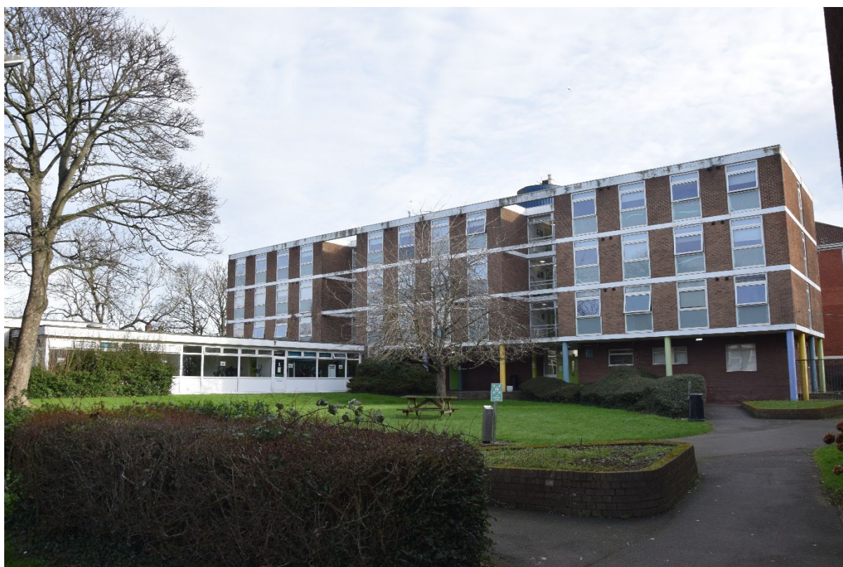
Photograph 26: 1960s accommodation block (DHW F), looking north-east
