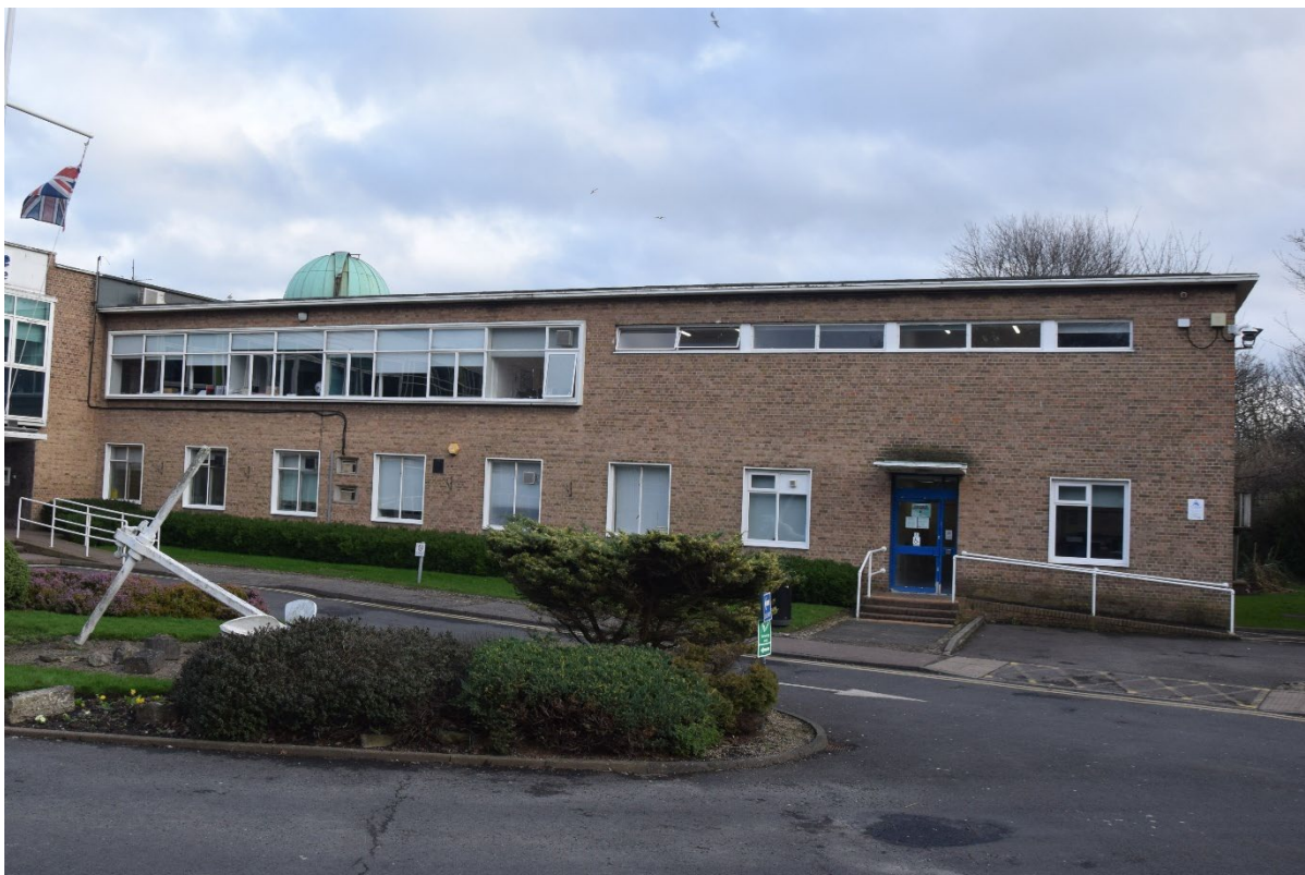
Photograph 1: The college administration building (western projection of the north end of Block A), looking south-east
