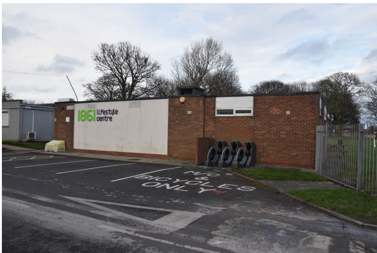
Photograph 38: Gymnasium, looking north-east
