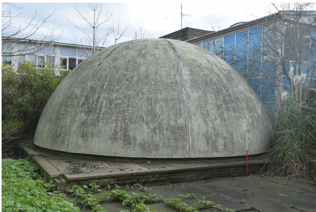
Photograph 12: The planetarium dome, looking south. The planetarium is now disused
