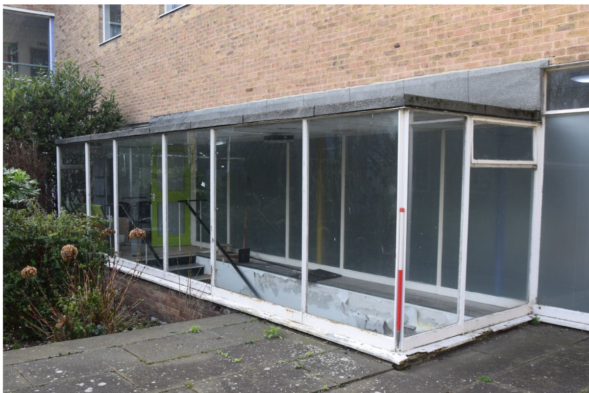
Photograph 43: Atrium of the planetarium, looking west
