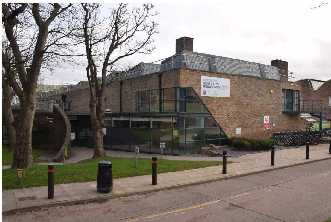
Photograph 22: Workshops (north end of Block F), looking south
