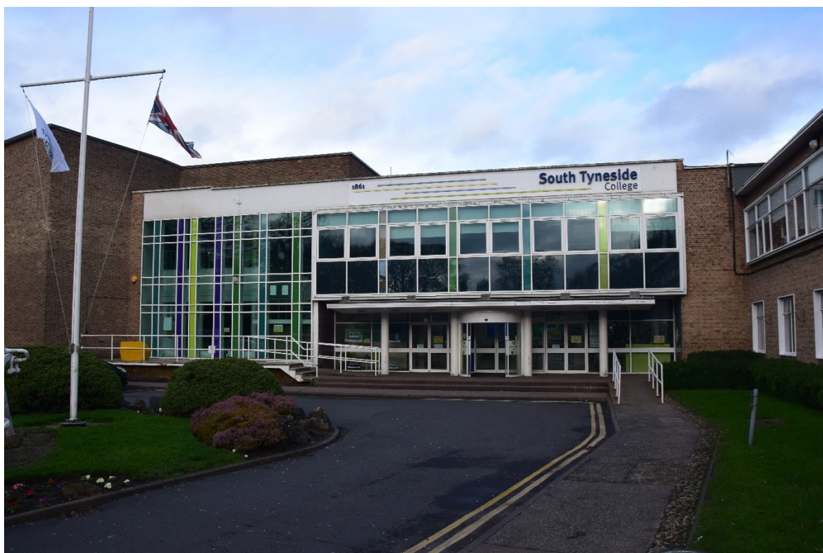
Photograph 8: Entrance Building (western side of Block B), looking north-east
