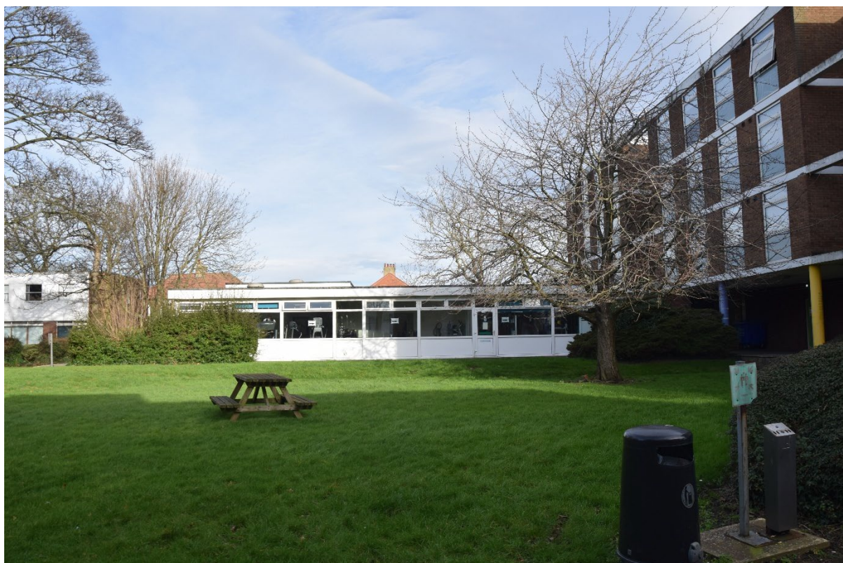
Photograph 27: 1960s accommodation block (DHW F), looking north
