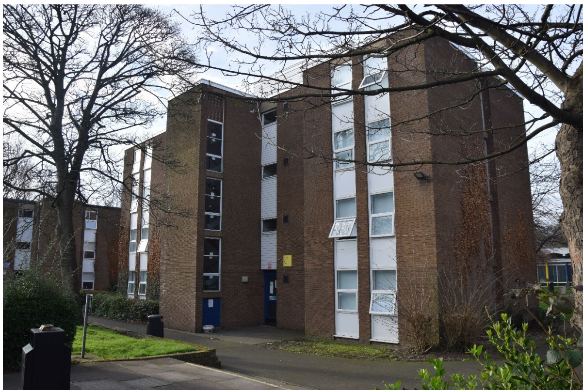
Photograph 35: Accommodation Block (DWH C), looking south
