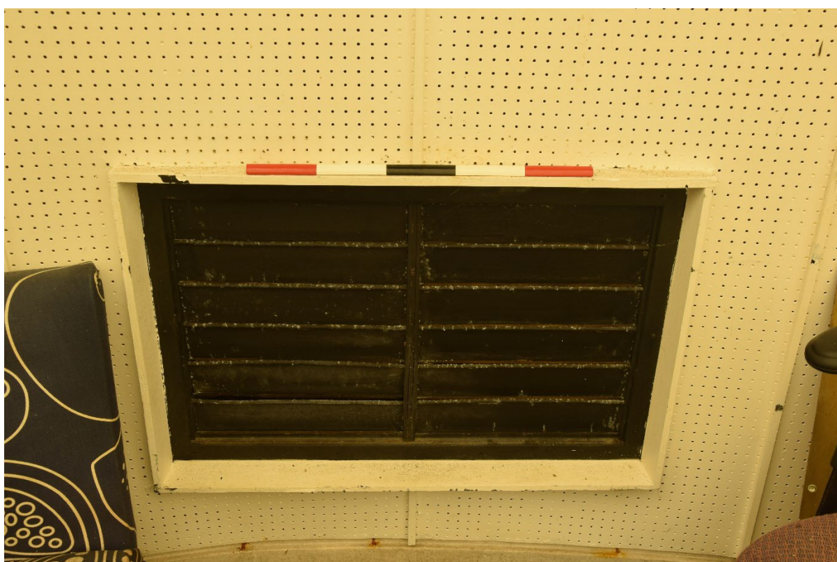
Photograph 56: Air vents in the west wall of the planetarium, looking south
