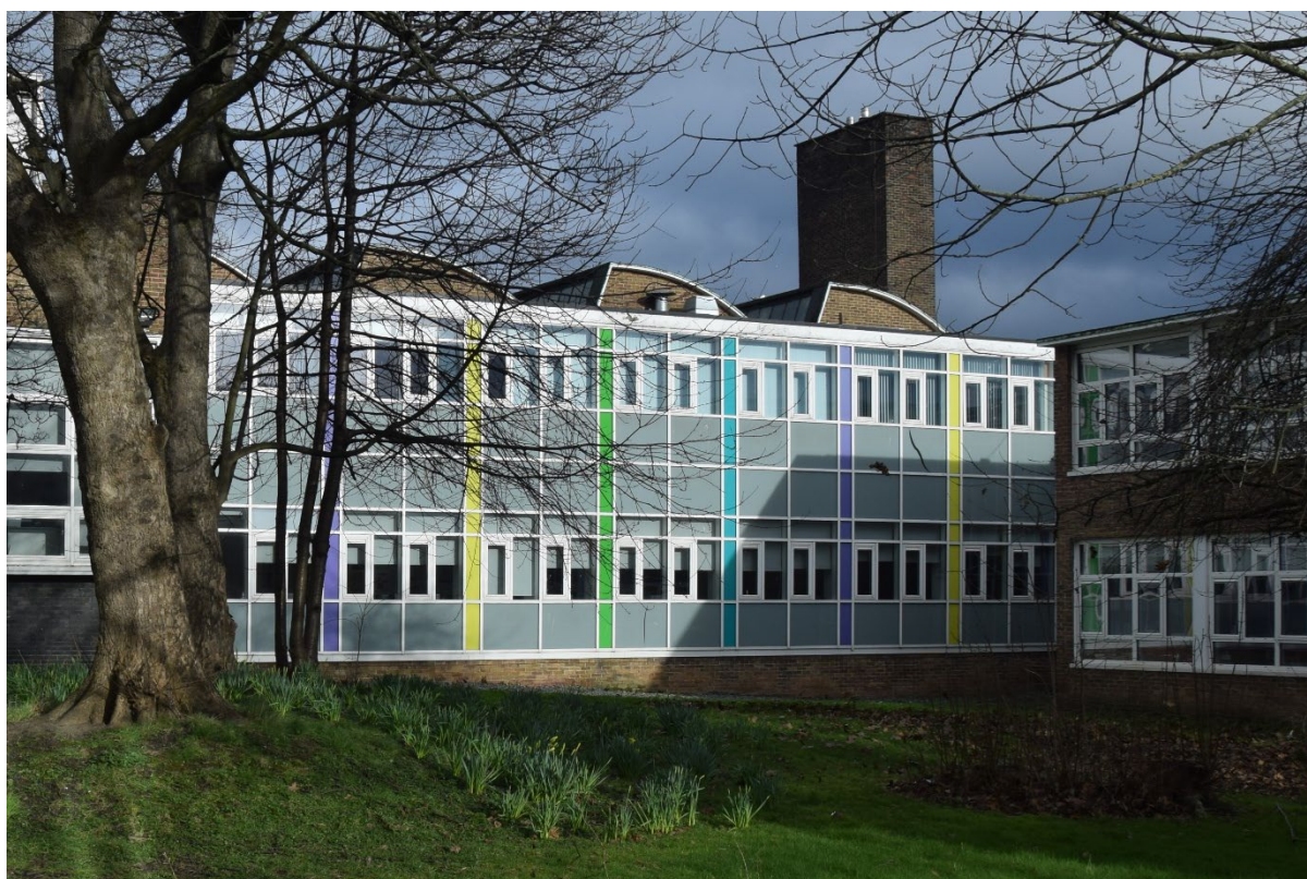
Photograph 20: Extension to the workshops (west face of the north end of Block E), looking east
