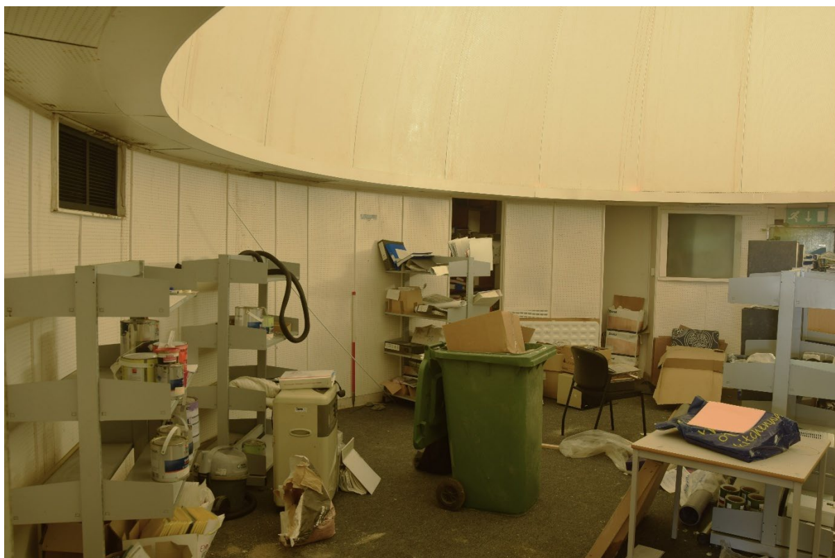
Photograph 49: East side of the planetarium, looking south-east
