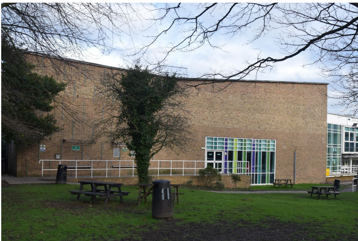
Photograph 10 (below): The communal building (western side of Block B), looking east
