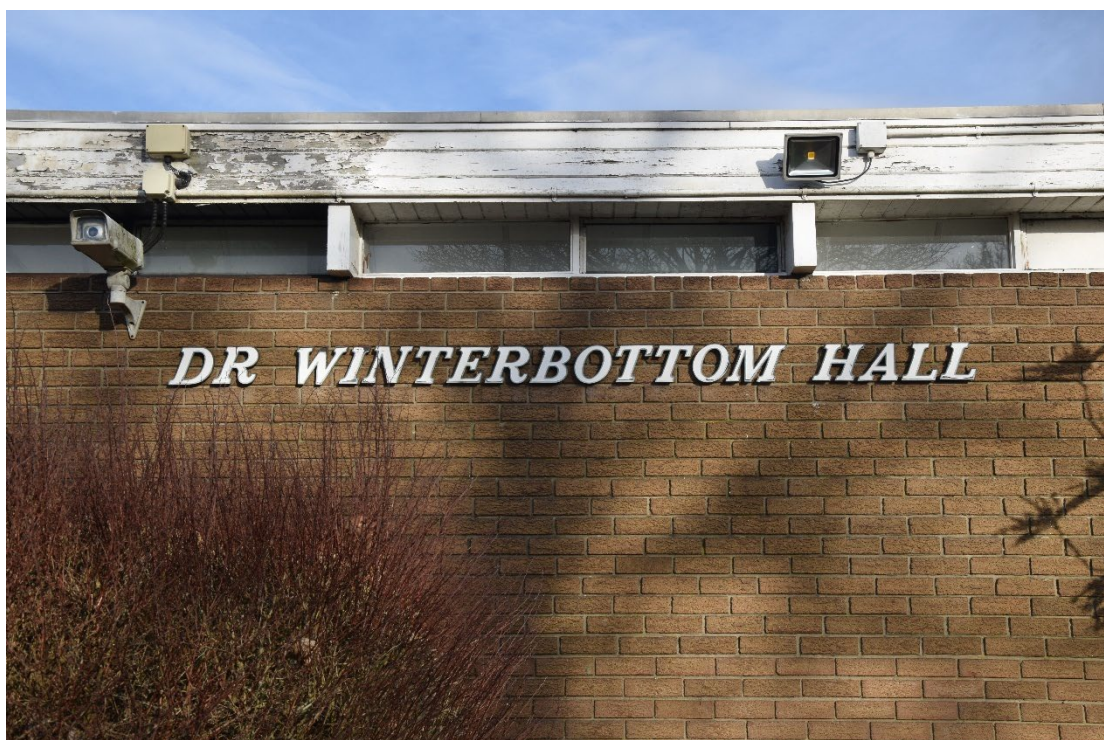
Photograph 30: Plaque on the side of the Dr Winterbottom Hall, looking north
