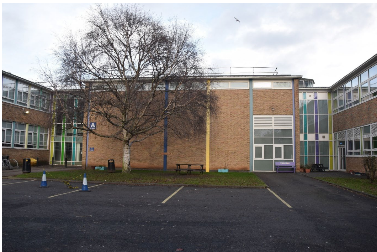
Photograph 13: Science Department (south end of Block A), looking north-east
