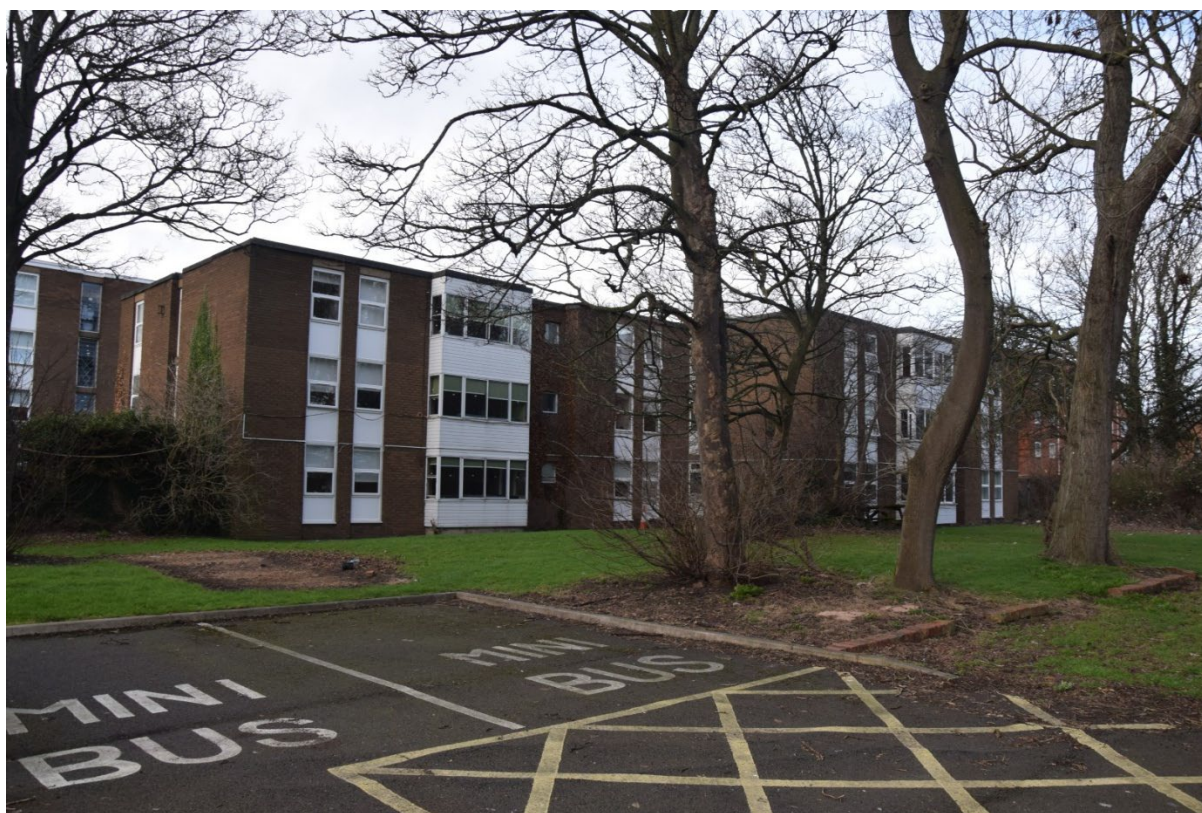
Photograph 36: Accommodation Block (DWH D-E), looking north-east
