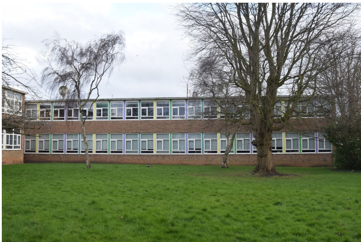
Photograph 7: Electrical and Radio Department (western projection of the centre of Block A), looking south-east
