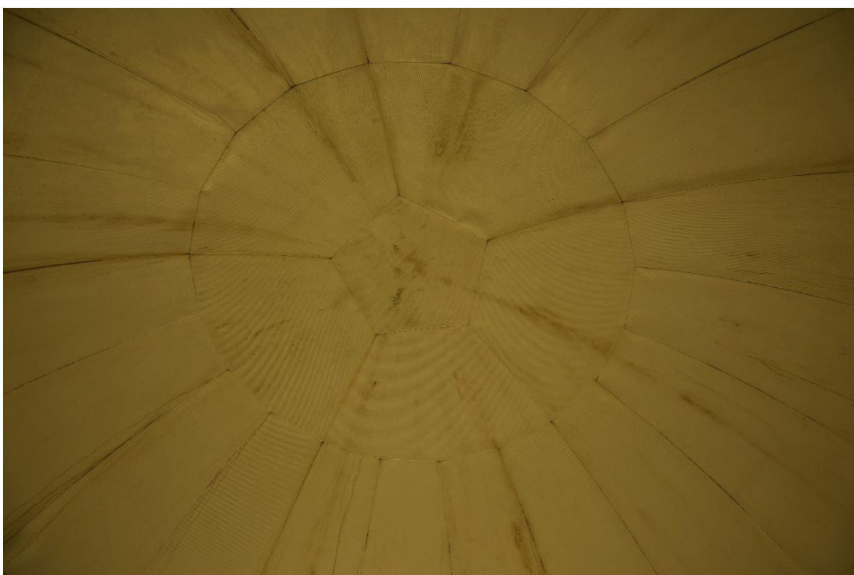
Photograph 52: View of the apex of the dome, looking south
