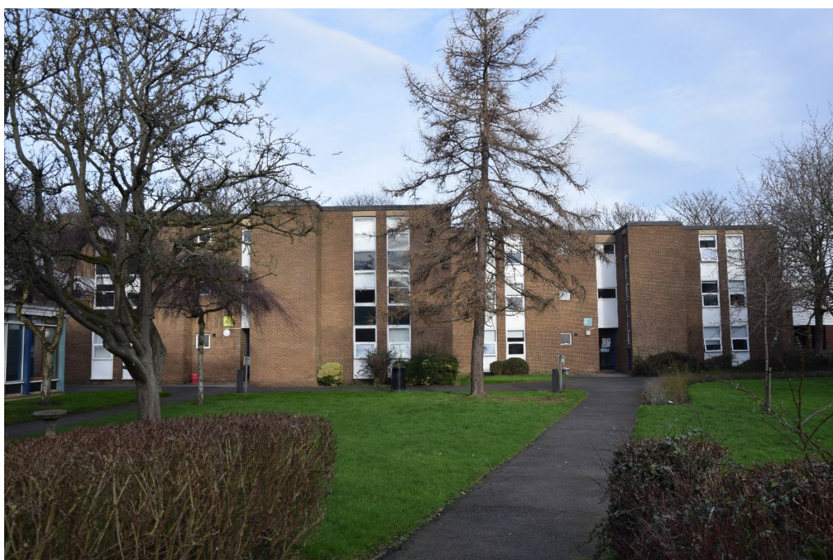
Photograph 34: Accommodation blocks (DWH A&B), looking north
