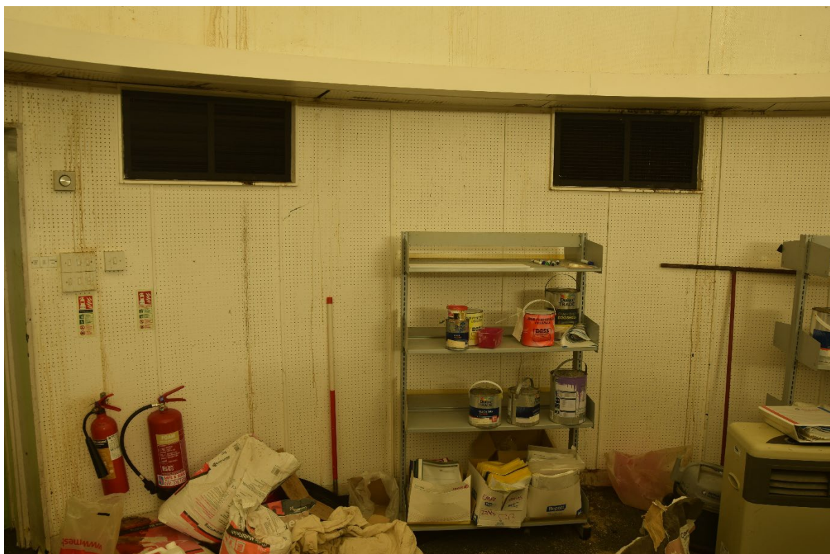
Photograph 55: Air vents in the east wall of the planetarium, looking north-east
