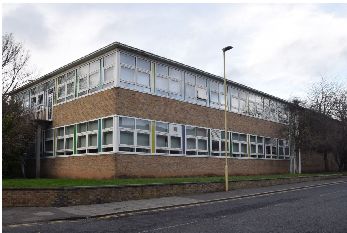
Photograph 14: Science Department (western projection of the south end of Block A), looking north
