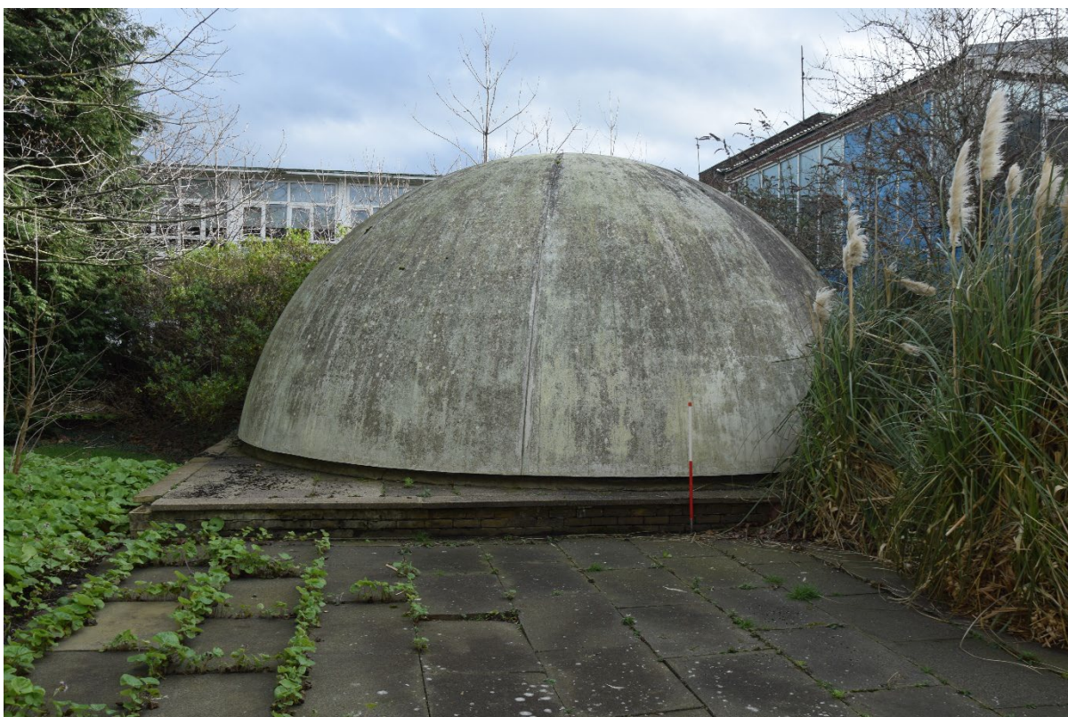
Photograph 39: Planetarium dome, looking south-east
